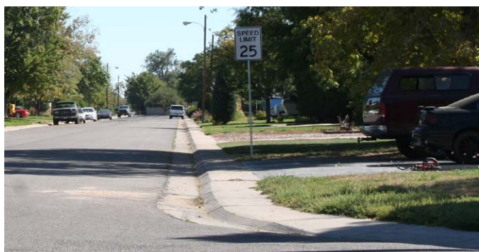
Narrow Attached Walk With Mountable Curb
