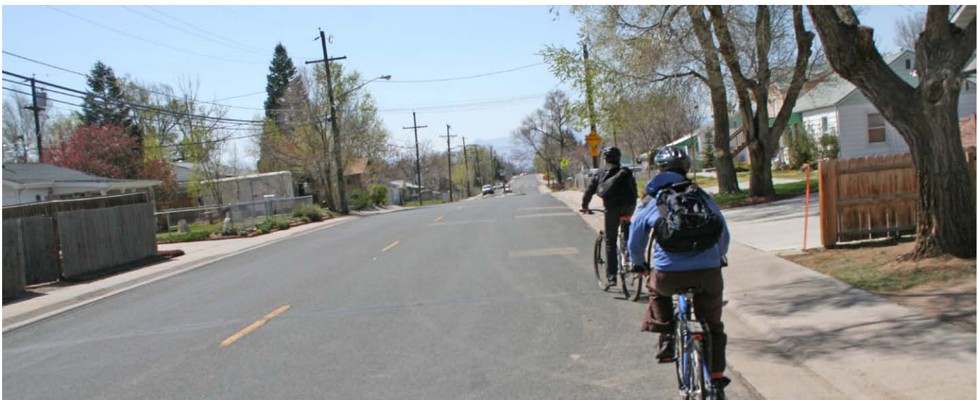
Typical Local Street in Historic City (Note Mountable Curb and Attached Sidewalk-60th Ave. at Olive Street)
