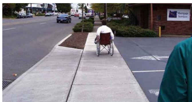
Separated Sidewalk Keeps Sidewalk Level At Driveways
